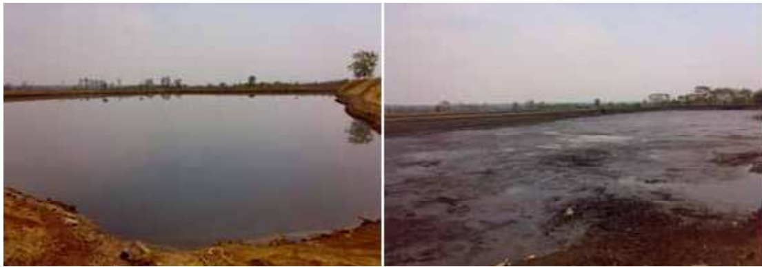
Figure 11: Anaerobic Lagoon in a Distillery in India ("The Global Methane Initiative", 2011)
